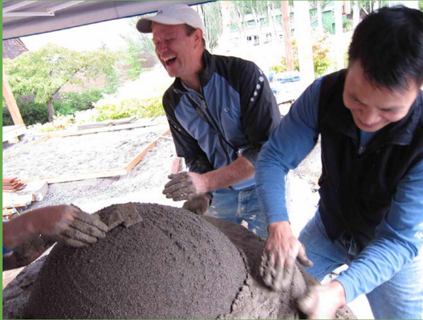
Constructed cob oven
